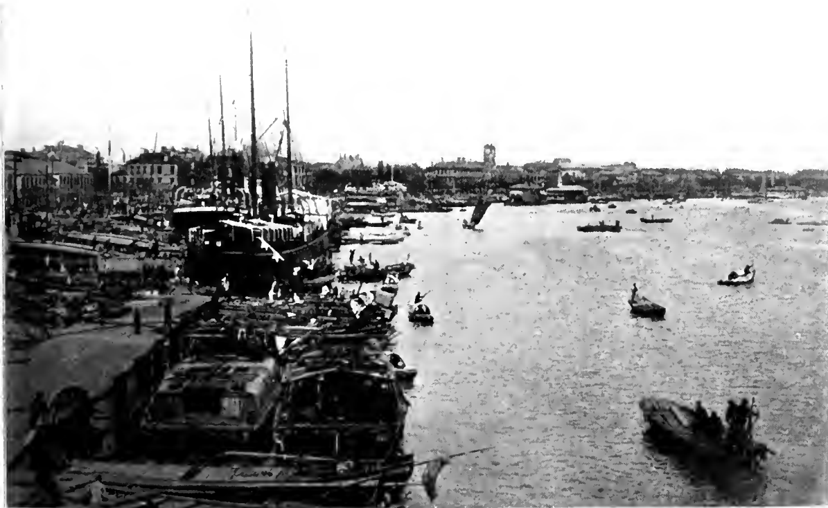
SHANGHAI: RIVER VIEW UP-STREAM
